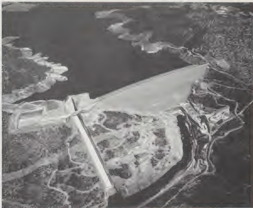
Figure 6.3 Oroville Dam on the Feather River in California. This is a 225 m (740 ft) tall earth dam with a volume of 61,000,000 m 3 (80,000,000 yd 3 ) (California Department of Water Resources).
