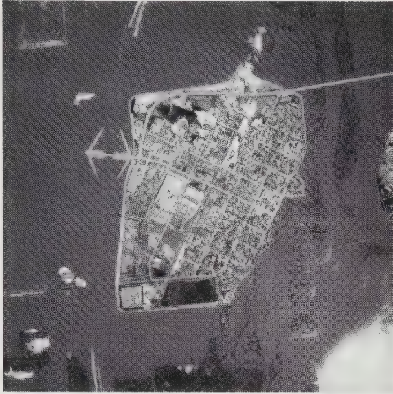
Figure 15.10 The town of Pembina, ND is located along the banks of the Red River. When the river reached flood stage in 1997, levees surrounding the town protected it from flooding. The normal river channel is barely visible on the right side of this aerial photograph. Interstate Highway 29, which is located outside the levees, is visible on the left. Part of the highway has flooded, but a bridge and ramps to the left of the town still extend above the water level. If the levees had not been built, most or all of the town would have been under water (U.S. Army Corps of Engineers - St. Paul District).
