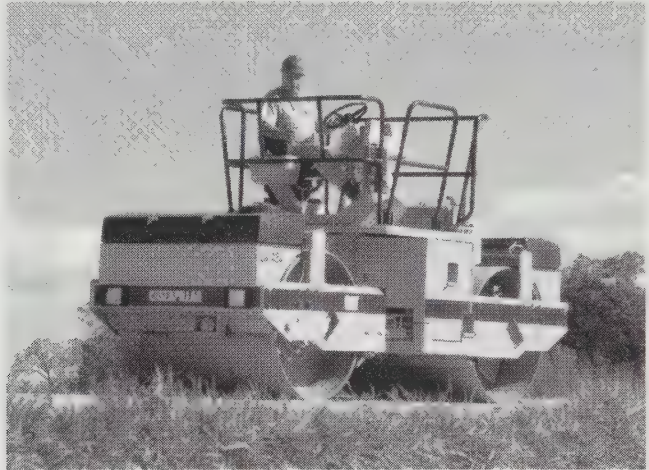
Figure 6.23 A smooth steel-wheel roller preparing to compact an asphalt pavement. (Caterpillar Inc.)
