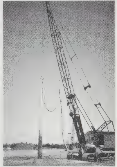
Figure 19.5 This crane is lowering a vibroflot into the ground (GKN Hayward Baker, Inc.).
