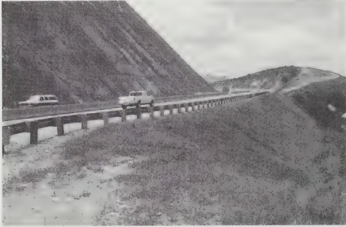
Figure 6.1 This four-lane highway was created by making a cut on the left side of the photo and in the background, and a fill in the foreground.
