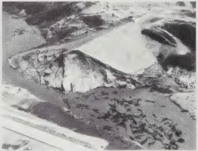
Figure 15.8 Teton Dam soon after failure. The reservoir was located to the left of the dam (U.S. Bureau of Reclamation).
