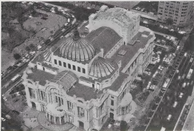
Figure 11.1 By 1950, the Palace of Fine Arts in Mexico City had settled about 3 m more than the surrounding streets.
