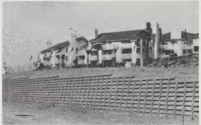
Figure 16.22 A crib wall.
