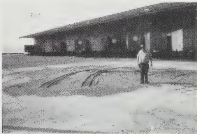
Figure 20.6 Sand boil at truck terminal in Port of Oakland, California, produced by the 1989 Loma Prieta Earthquake. (Earthquake Engineering Research Center Library, University of California, Berkeley, Steinbrugge Collection)
