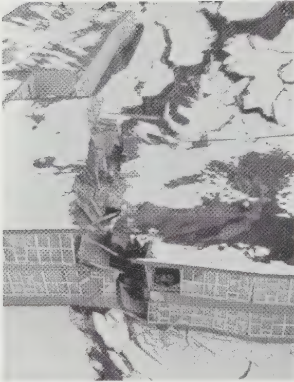
Figure 20.18 The head scarp of this landslide, which was triggered by the 1964 Alaska Earthquake, extended beneath the Government Hill Elementary School in Anchorage. The building split apart and dropped about 2.8 m (9 ft). (Earthquake Engineering Research Center Library, University of California, Berkeley, Steinbrugge Collection)
