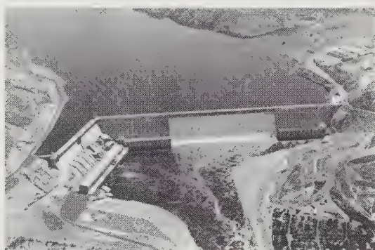
Figure 15.1 Grand Coulee Dam on the Columbia River in Washington. This is one of the largest concrete gravity dams in the world (U.S. Bureau of Reclamation).
