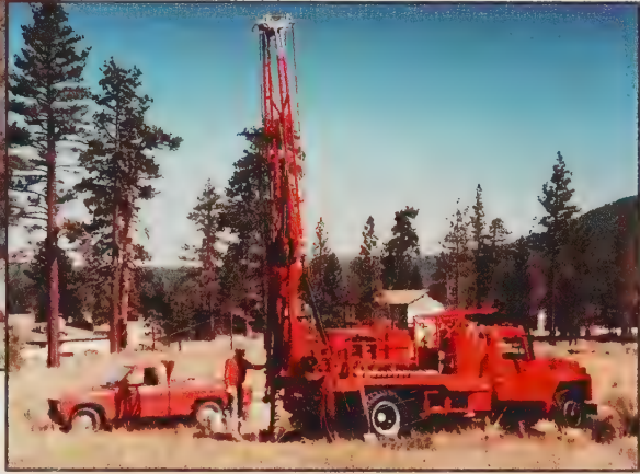
▼ Plate J Drilling an exploratory boring
