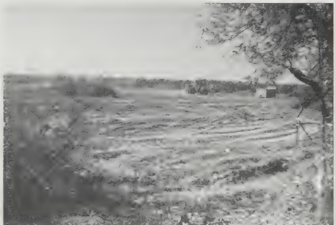
Figure 6.10 Clearing and grubbing in a former orange grove. The trees are being removed and hauled to the dumpster seen in the background.
