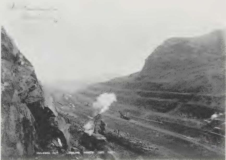
Figure 6.4 Construction of the Culebra Cut for the Panama Canal, 1907. The steam-powered excavators placed loads of soil and rock into railroad cars that hauled them away (Library of Congress).
