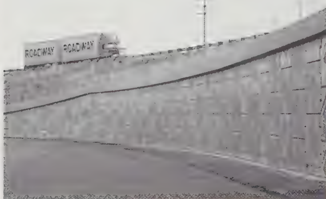
Figure 16.27 A completed reinforced earth wall (The Reinforced Earth Company).
