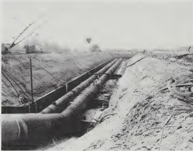
Figure 8.28 This 11 m (35 ft) deep excavation was required to construct these two water supply pipelines. The excavation extends 10 m (35 ft) below the groundwater table, and a river is located just beyond the excavation on the left side of the photograph. Therefore, a temporary dewatering system has been installed to draw down the groundwater table. This system includes a series of pumped wells, including the one in the right foreground (Photo courtesy of Foothill Engineering).
