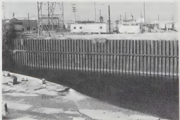
Figure 16.23 A sheet pile wall.
