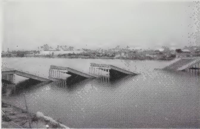
Figure 20.17 The Showa Bridge in Niigata, Japan, collapsed due to the formation of lateral spreads in the underlying soils during the 1964 earthquake. The lateral spreads moved the piers out of position, thus removing support from the simply supported deck. (Earthquake Engineering Research Center Library, University of California, Berkeley, Steinbrugge Collection)
