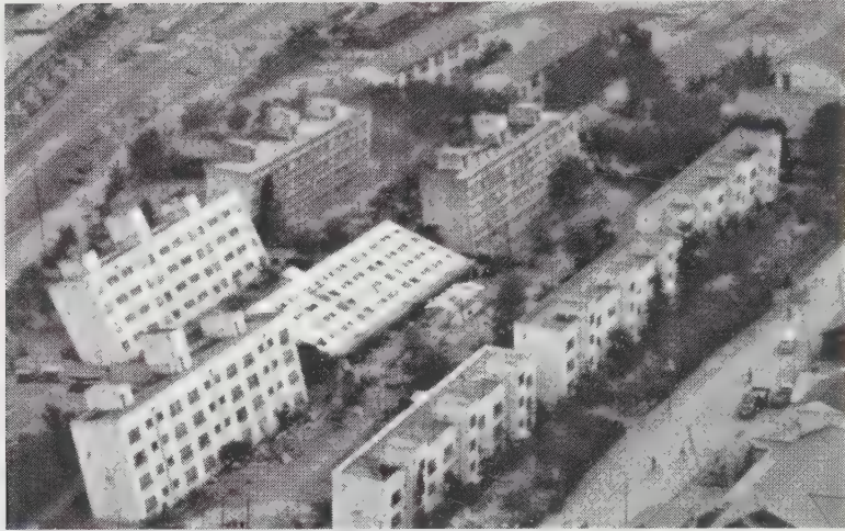
Figure 20.9 The soils below these apartment buildings in Niigata, Japan, liquefied during the 1964 earthquake, which produced bearing capacity failures (as discussed in Chapter 17). The failure reportedly occurred very slowly, and the buildings were very strong and rigid, so they remained virtually intact as they tilted. There was very little damage to the interior, and the doors and windows still functioned after the failure. Afterwards, the occupants of the center building were able to evacuate by walking down the exterior wall. (Earthquake Engineering Research Center Library, University of California, Berkeley, Steinbrugge Collection)
