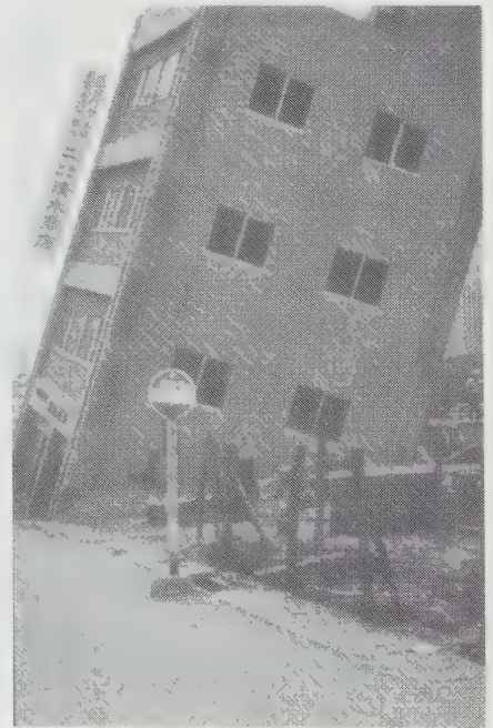
Figure 20.10 The soils below this building in Niigata, Japan, liquefied during the 1964 earthquake, causing settlement and bearing capacity failures. (Earthquake Engineering Research Center Library, University of California, Berkeley, Steinbrugge Collection)
