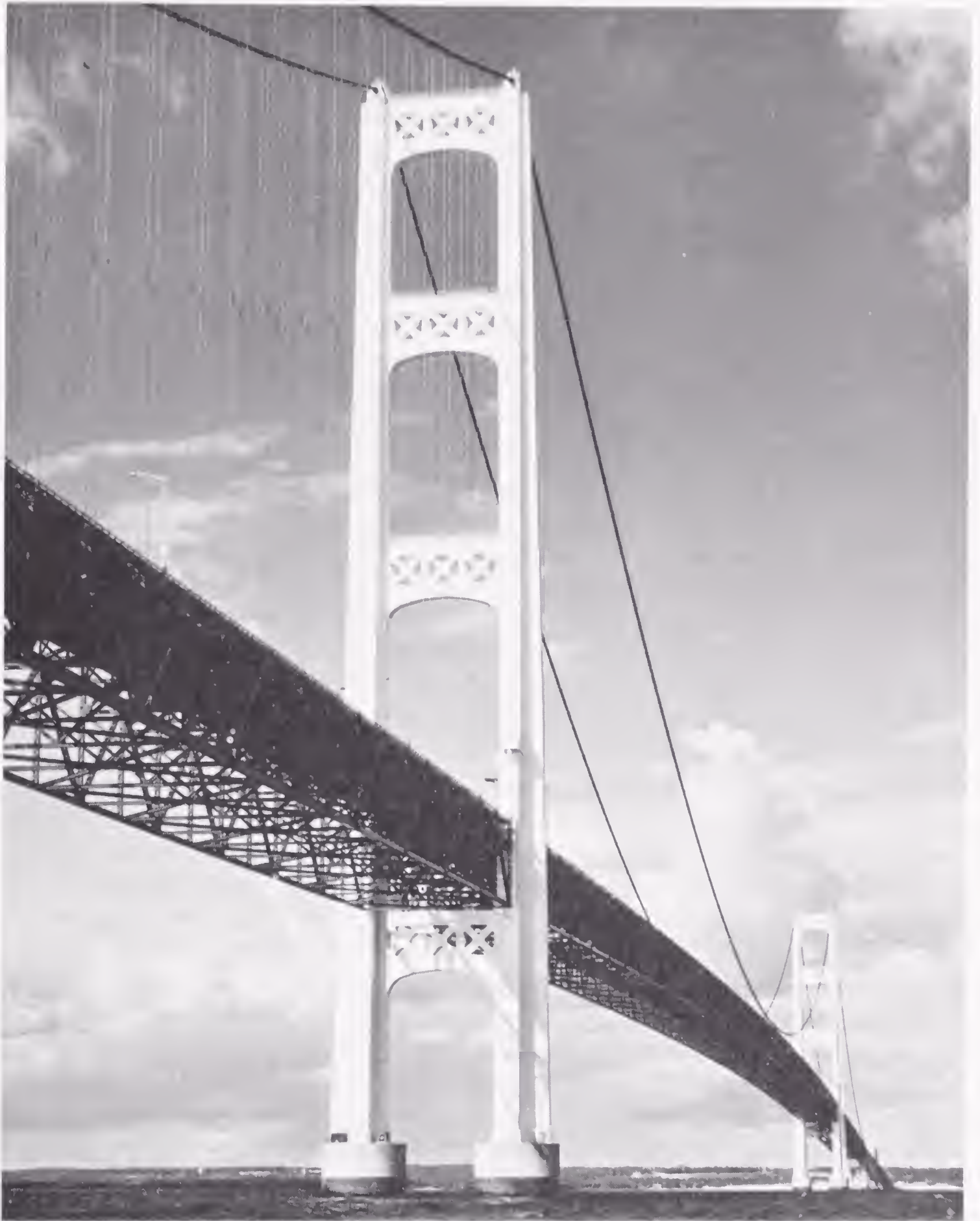
Figure F.4 Mackinac Straits bridge, Michigan. Longest suspension bridge, anchorage to anchorage, 8,614 ft; third longest main span, 3,800 ft (Photograph furnished and reproduced by courtesy of the designer, the late Dr. D. B. Steinman, Consulting Engineer, New York)
