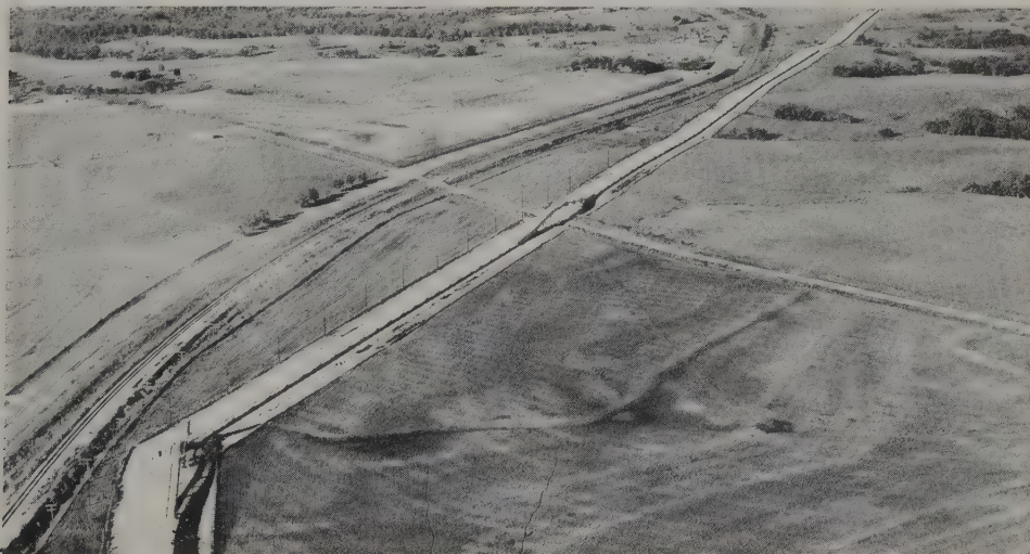
Figure 5.39. Five-and-one-half-mile overland conveyor.
