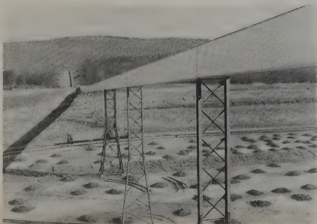
Figure 5.35. Conveyor in enclosed gallery.
