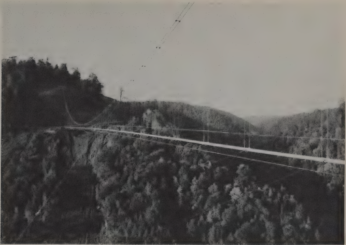
Figure 5.17. Savage River pipeline.
