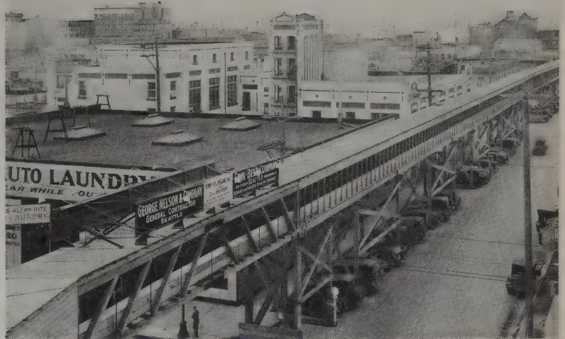
Figure 5.38. Denny Hill conveyor system.
