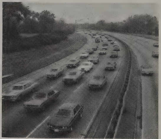
Figure 16.6. Level of service E as viewed looking up stream on a typical freeway indicating unstable flow, lower operating speeds than level D and some momentary stoppages. SOURCE: Illinois Department of Transportation.
