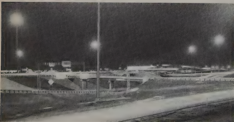
Figure 20.4. High-mast lighting installation in Dallas. SOURCE: Texas Highway Department.
