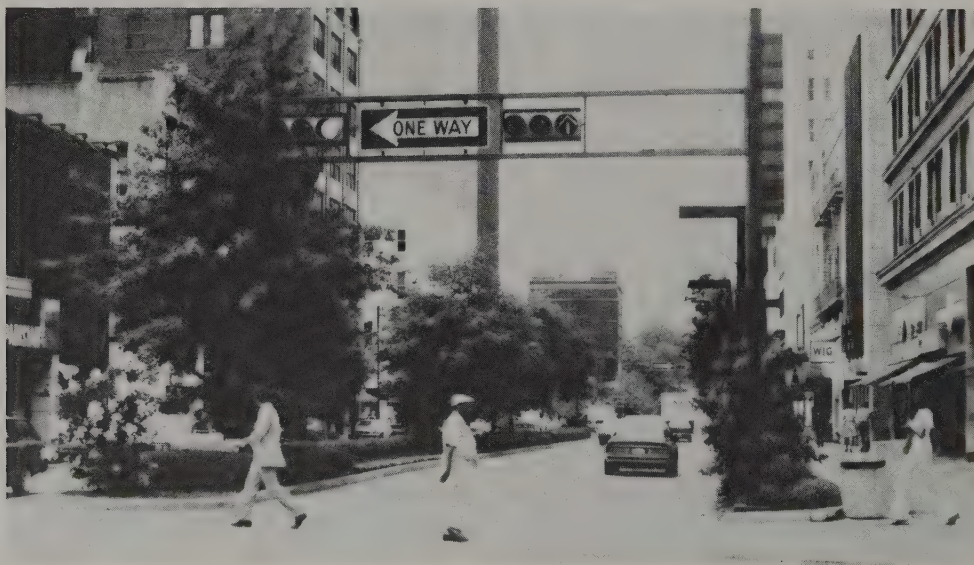
Figure 13.25. Traffic signal and information signs mounted in space frame. SOURCE: Traffic Planning Associates, Inc.
