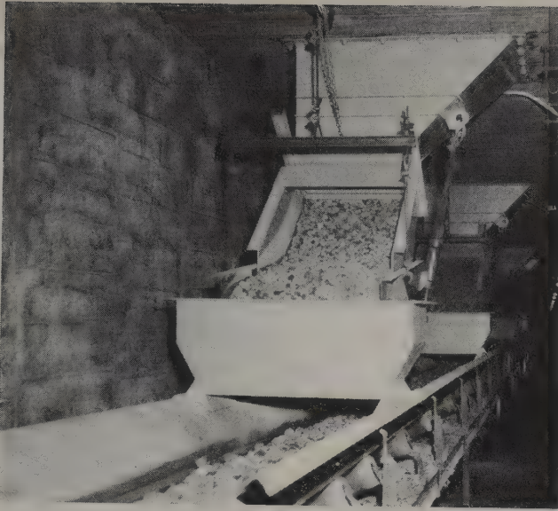
Figure 5.26. Multiple feeders in tunnel.
