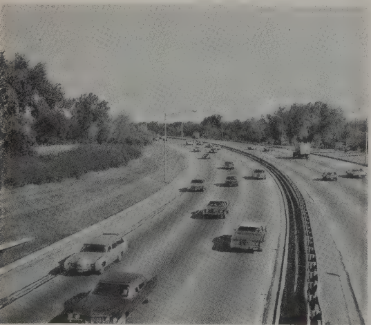
Figure 16.4. Level of service C as viewed looking up stream on a typical freeway indicating stable flow, higher volume, and more restrictions on speed and lane changing. SOURCE: Illinois Department of Transportation.
