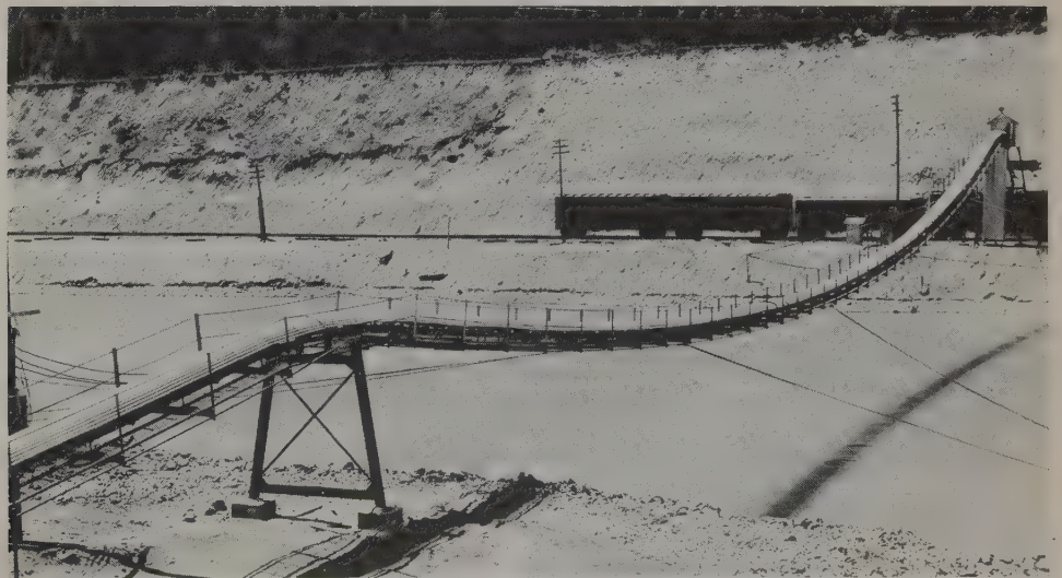
Figure 5.23. Cable-suspended support across river.
