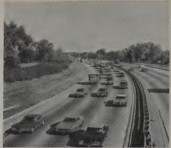
Figure 16.5. Level of service D as viewed looking up stream on a typical freeway indicating approaching unstable flow, little freedom to maneuver, and condition tolerable for short periods. SOURCE: Illinois Department of Transportation.
