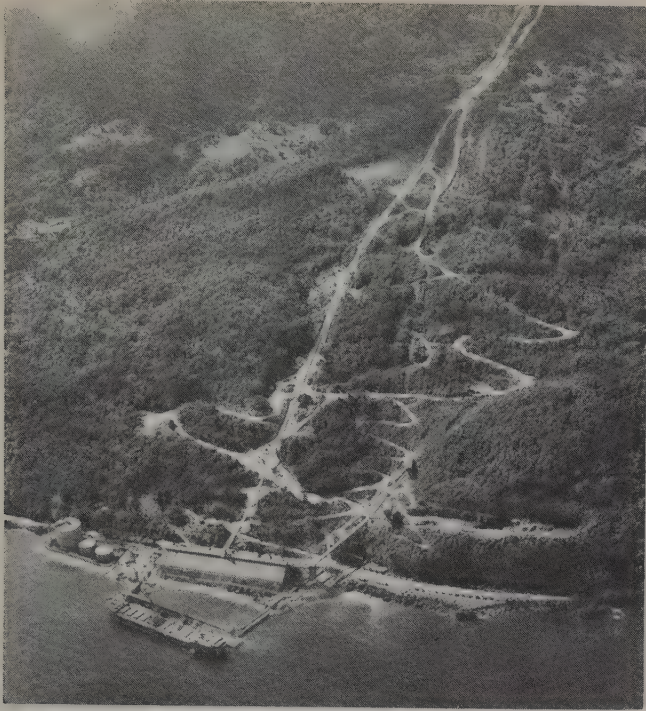
Figure 5.41. Six-and-one-half-mile conveyor system.
