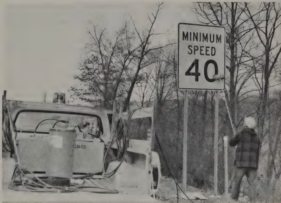
Figure 23.5. Typical sign washing equipment and operation. SOURCE: Pennsylvania Department of Transportation, Bureau of Traffic Engineering, Harrisburg, Pa.
