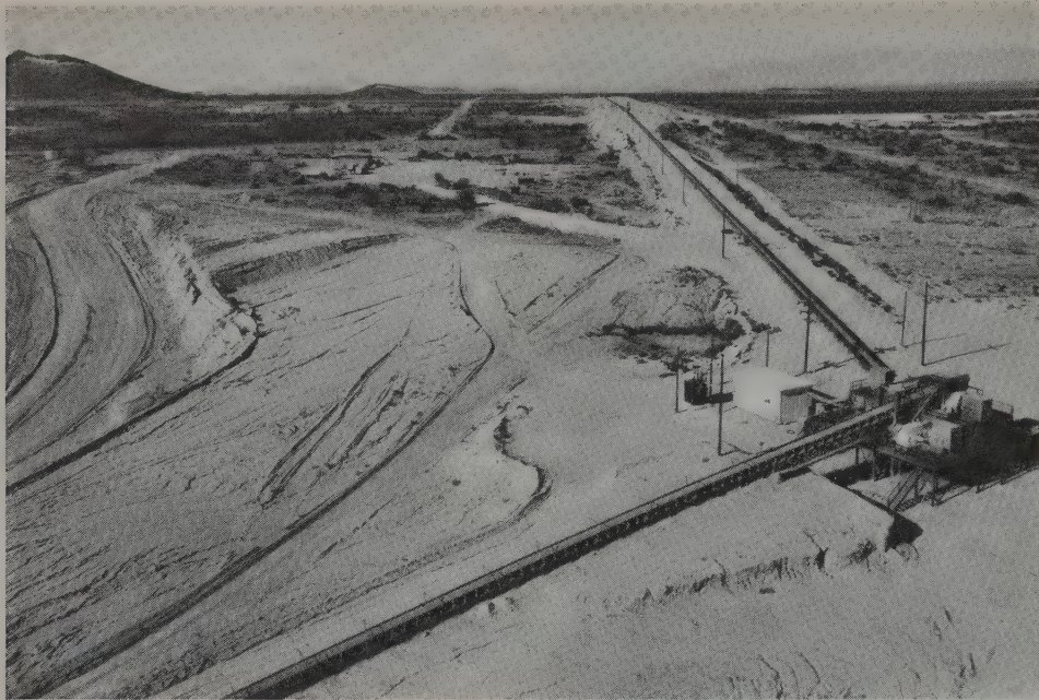
Figure 5.43. High-capacity conveyor system.
