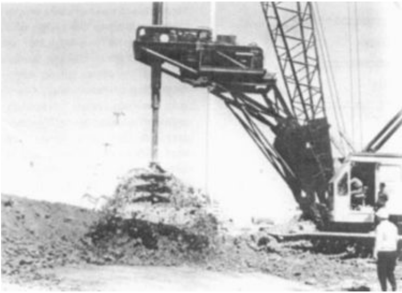
FIGURE 13.2. Crawler-mounted drilling machine spinning soil from auger after removal from shaft being excavated to diameter of 4 ft.
