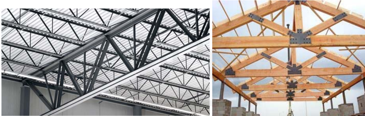
Figure 1-5: Steel and timber trusses
