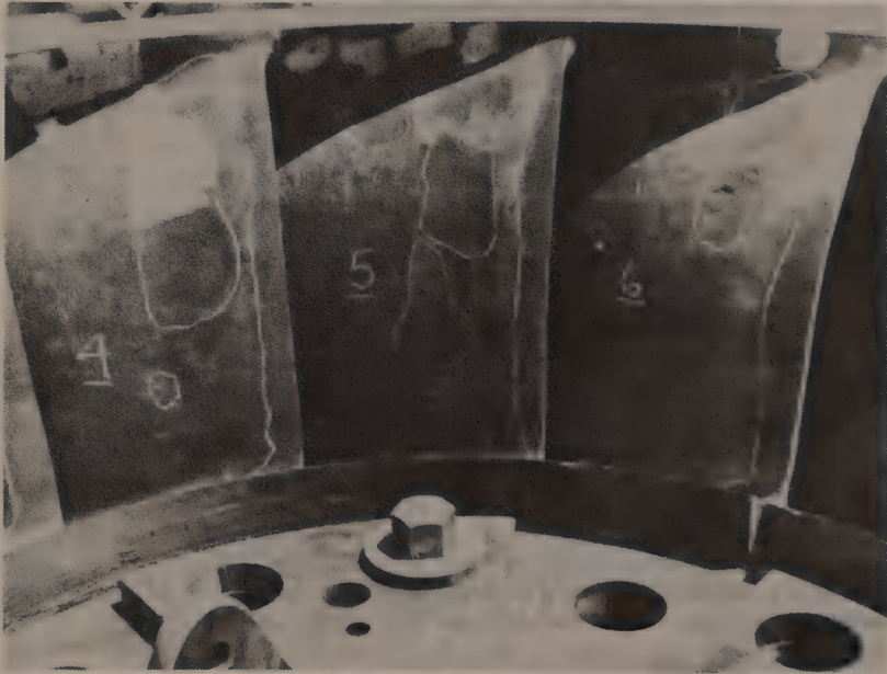
Figure 16.17 Cavitation pitting of Francis wheel and scroll case at Mammoth Pool Powerhouse after 2\frac{1}{2} yr of operation. Conditions of service were relatively severe. Turbine rating: 66,000 kW at effective head of 290 m; operating speed 360 rpm. The bright shiny areas are stainless-steel welds that have withstood cavitation pitting for over a year. (Courtesy of Southern California Edison Co.)
